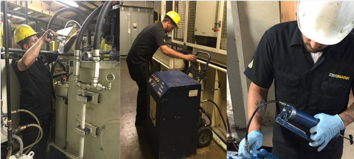
Zimmark Service Technician Oil Sampling, Oil Decontaminating and Greasing
